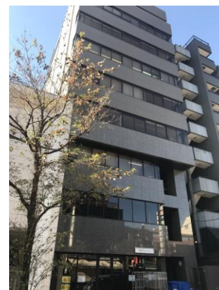
Commercial, office and residential building in Kagurazaka 6-Chome
